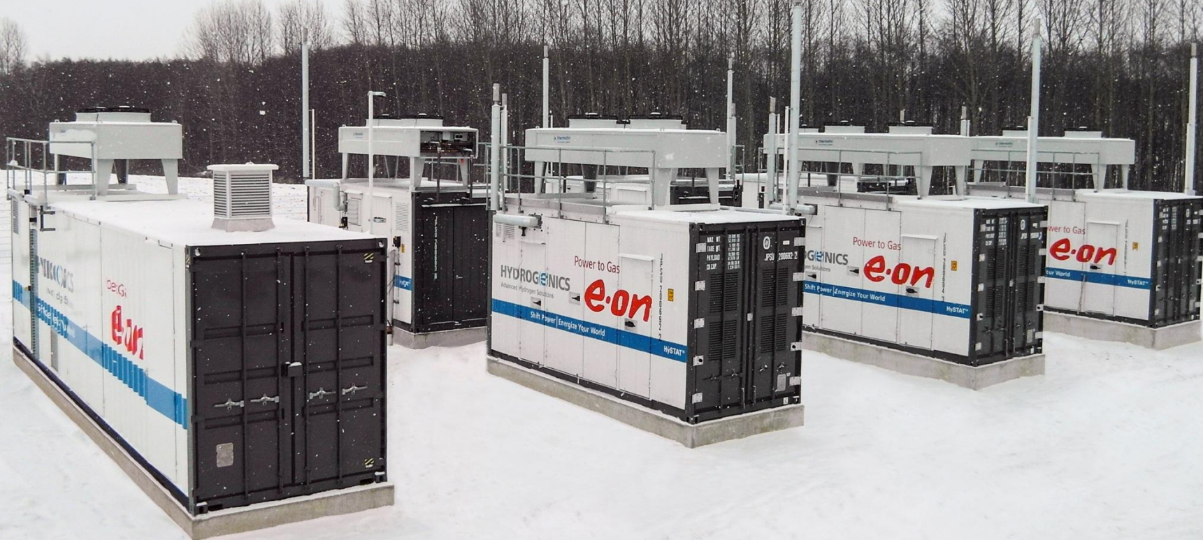
2 MW – 360 Nm 3 /h 'Power To Gas' Hydrogen feed in to HP natural gas line E.On Falkenhagen
