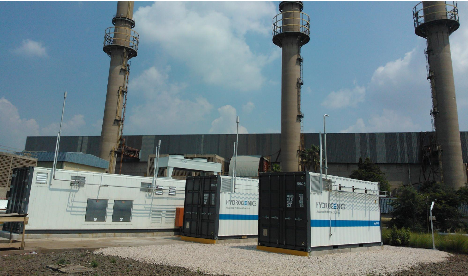
South Africa – 2 X 60 Nm 3 /h + H 2 and O 2 compression – industrial gas
